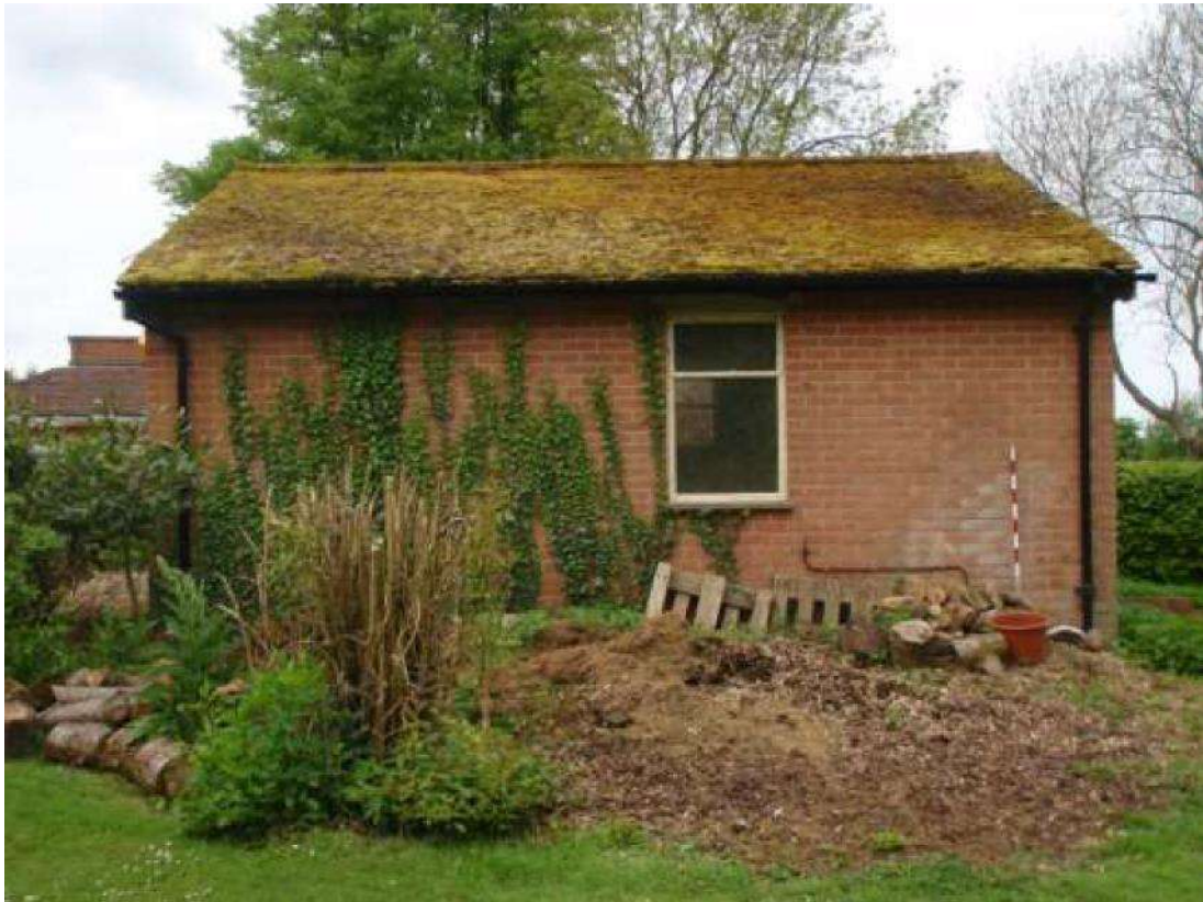
Plate 13: Side view of the garage (facing SW)
