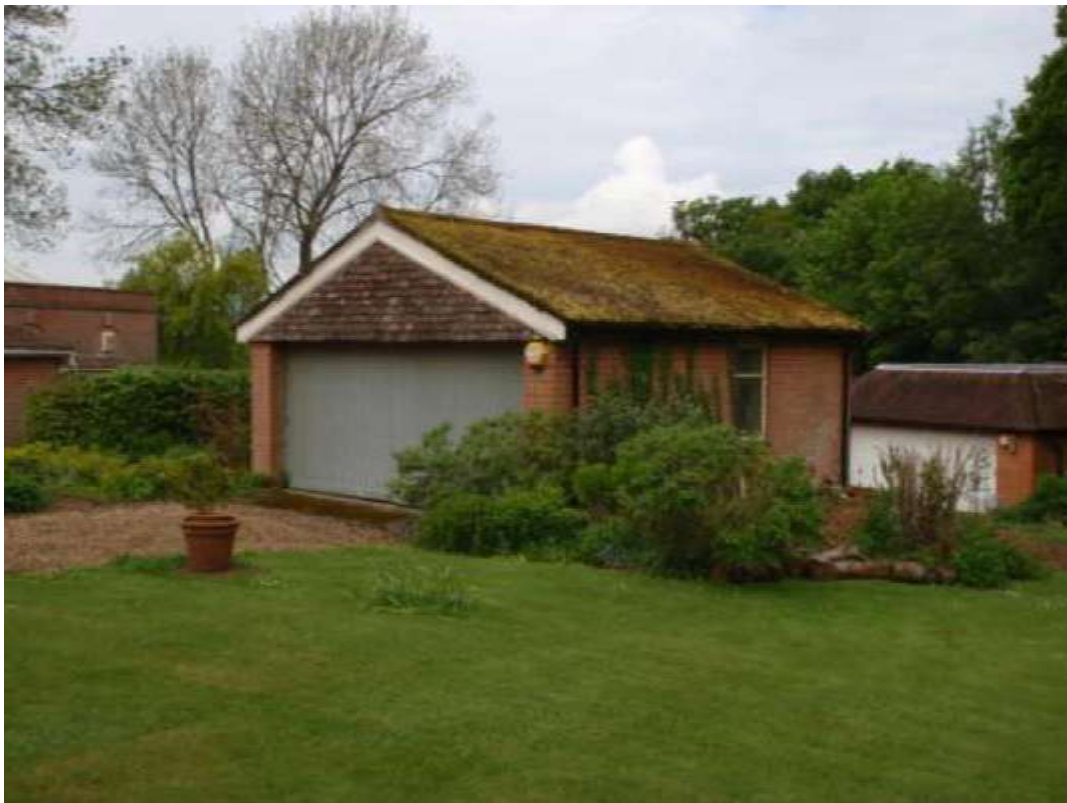
Plate 11: View of garage to be demolished (facing WNW)
