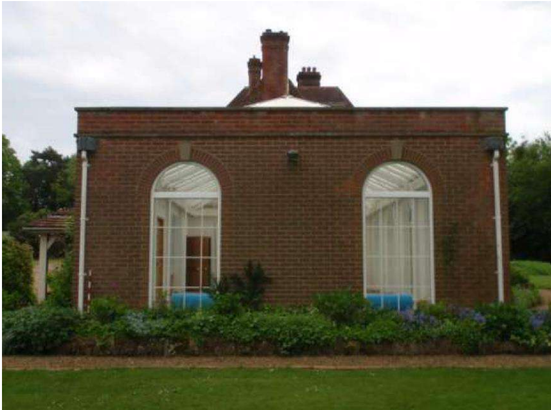
Plate 18: View of the pool house (facing SE)
