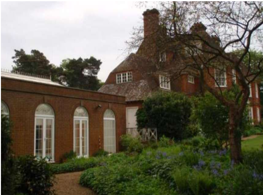
Plate 19: View of the pool house and main house (facing ESE)
