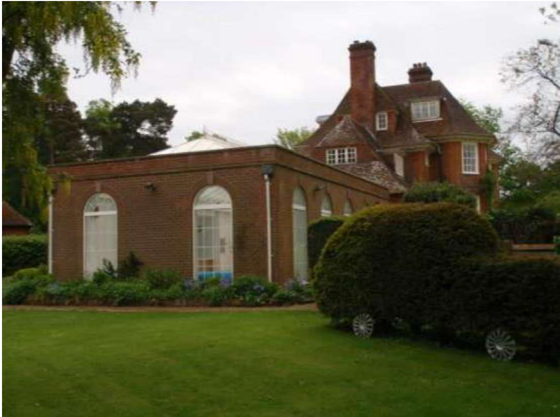
Plate 20: View of the pool house (facing SE)
