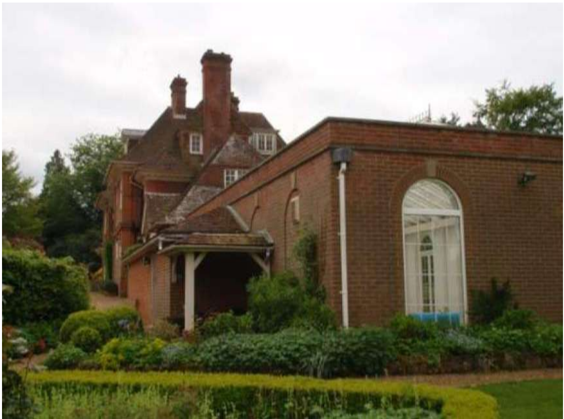
Plate 21: View of the pool house (facing SSE)
